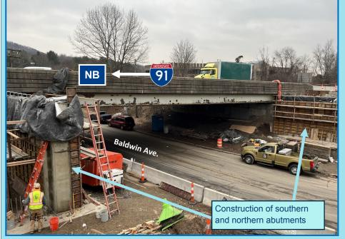
As part of the improvements, I-91 NB will be widened to provide an additional lane from the merge of the Exit 1A ramp to the rest stop in Middletown. When widening interstates and other roadways, bridges over or under local roads must be widened as well. By December, work progressed with widening of the I-91 NB bridge over the local road, Baldwin Avenue (see C the location of this site in the map above ).
